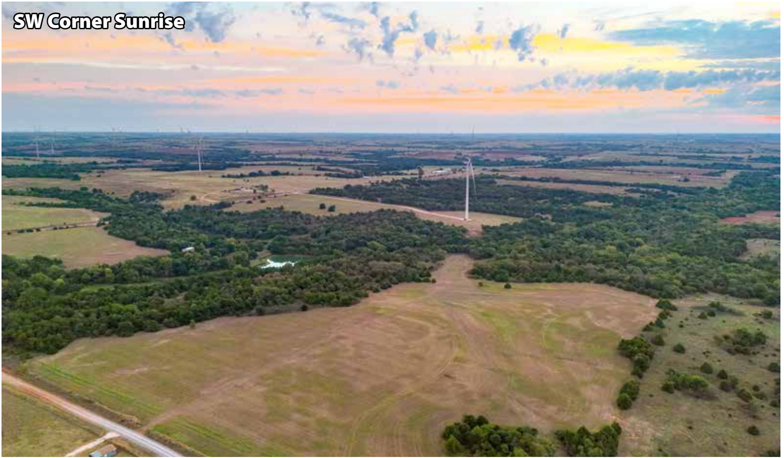
SW Corner View
