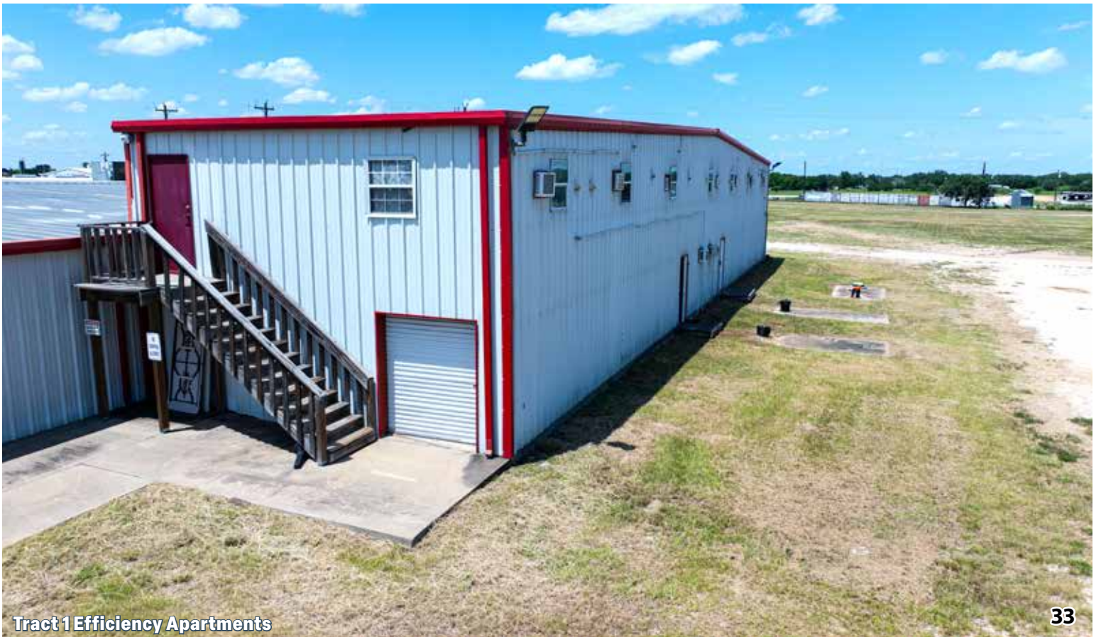
Tract 1 Additional Storage Building
