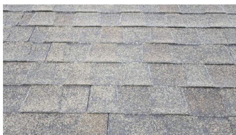
Significant granular loss
