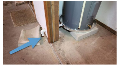
Improper termination
