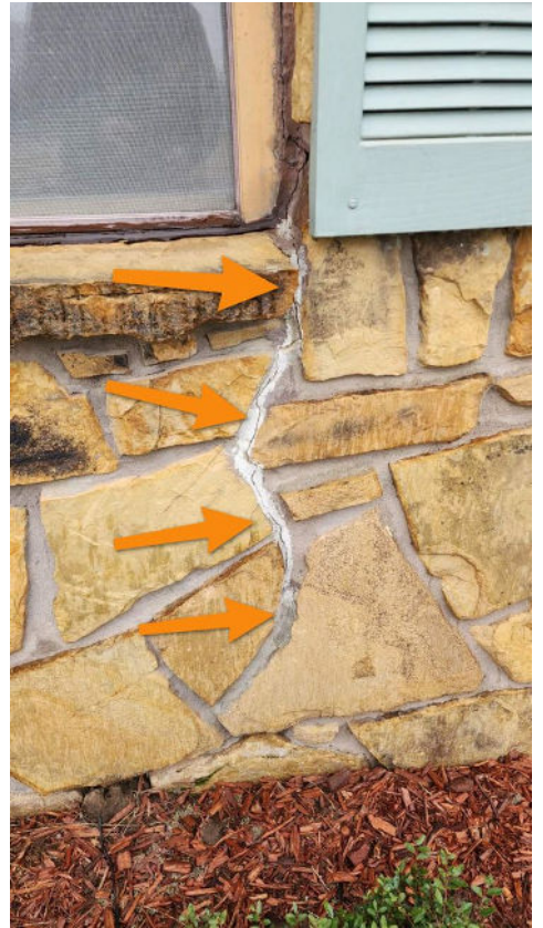
Right side under window
