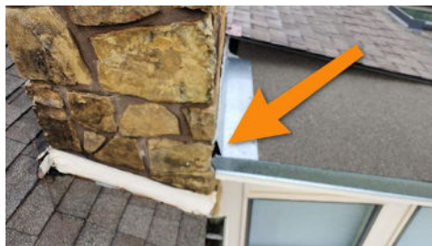
Base of chimney
