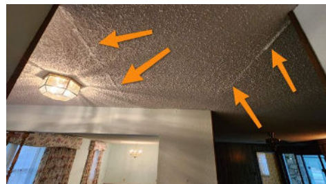
Entry/seam cracking
