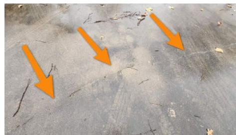
Driveway cracks
