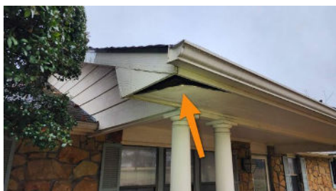
Covered front porch
