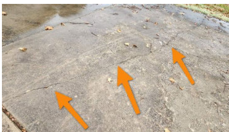
Driveway cracks
