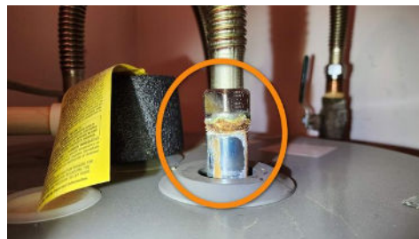
Corrosion noted
