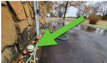
Sewer clean out location
