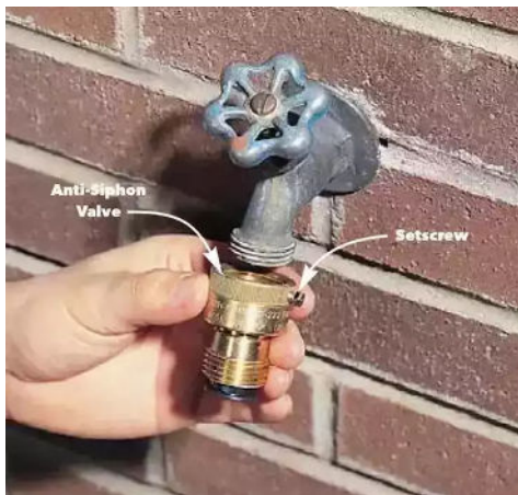
Example of Anti-Siphon Device
