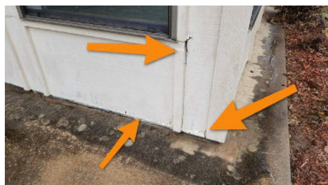
Sun room siding
