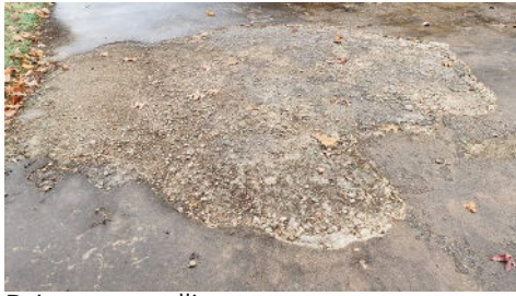
Driveway spalling
