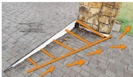
Recommend build up to divert water
