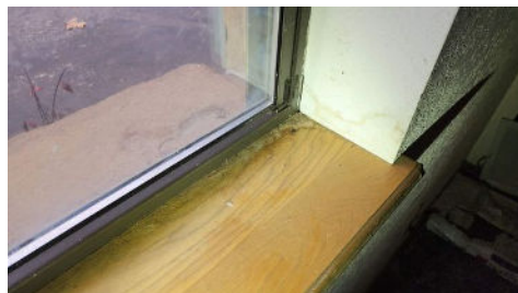
Room left of garage
